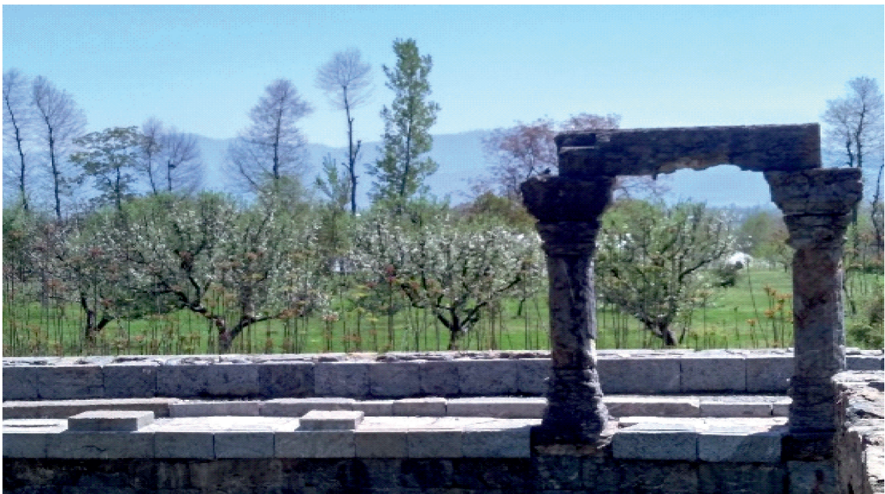
Figure 11: Photo captured by Uman Riyaz on 17 April 2017 of two columns (part of padkshina path) in Martand Sun Temple
