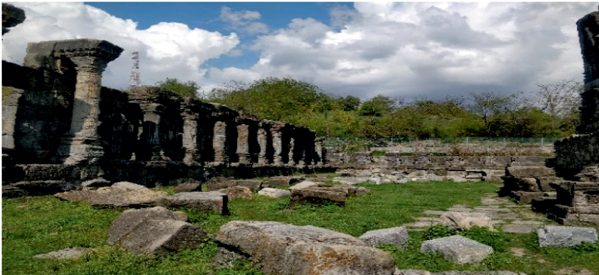
Figure 13: Photo captured by Uman Riyaz on 21 April 2020 inside the Martand Sun Temple represents continuation disorganization of work
